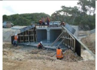
The Dry Creek Box culvert with the seaward wing walls poured. On top Engineers Nario Brown, Keith Tangwata and Makau Kalsakau assisted by Subu Kaldang set out the reinforcing for the headwall, while workers below fill scour protection reno mattresses with rocks.
